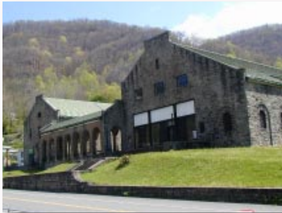
Pocahontas Coal Company Store and Offices, Itmann, Wyoming County.
