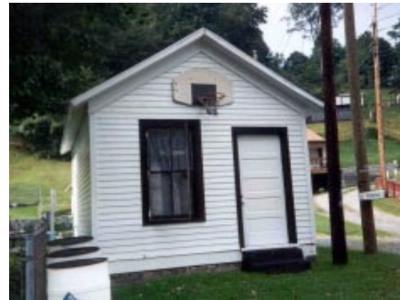
Former Coopers Post Office, Mercer County.
